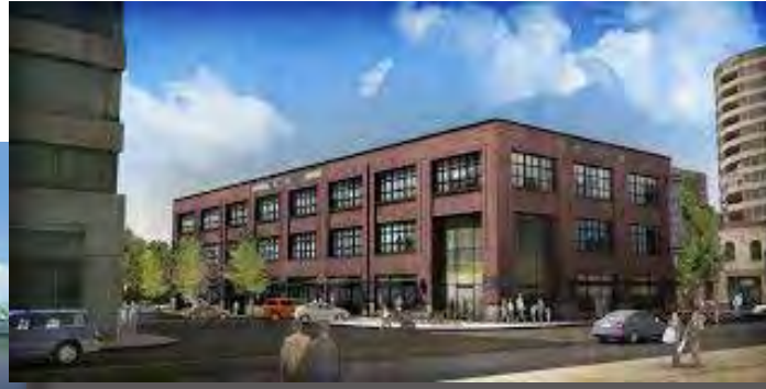
The Hudson Building
