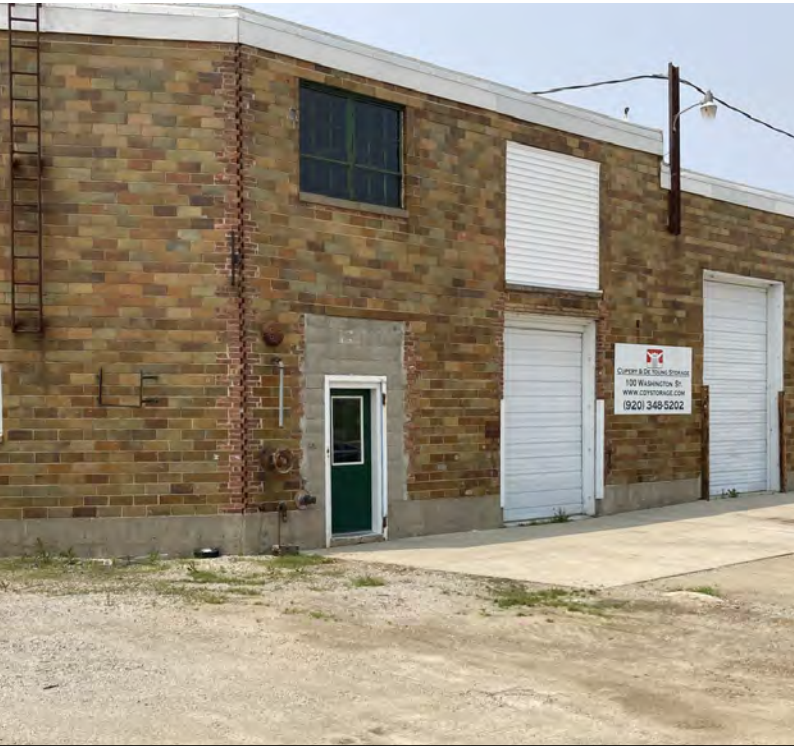
Exterior of Building
