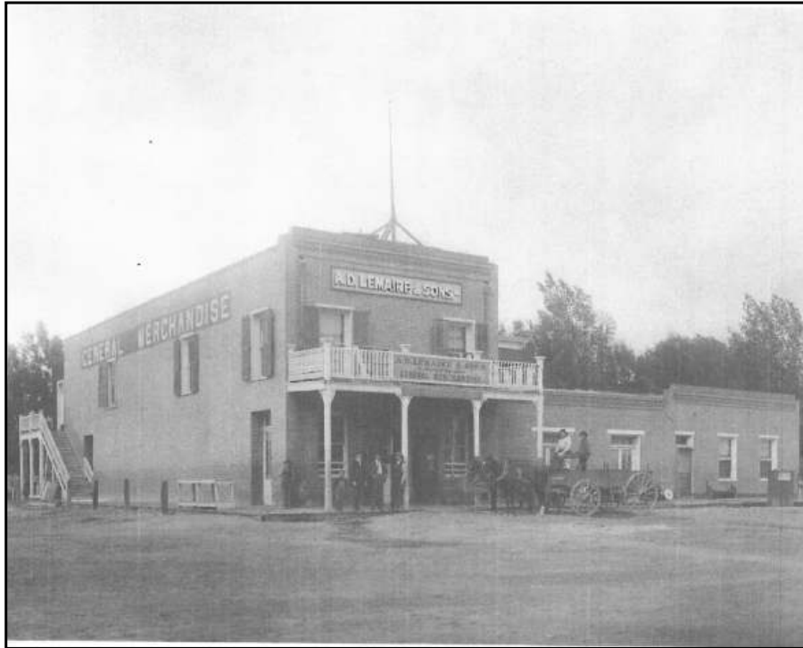
25 : Historic photograph of building exterior.
