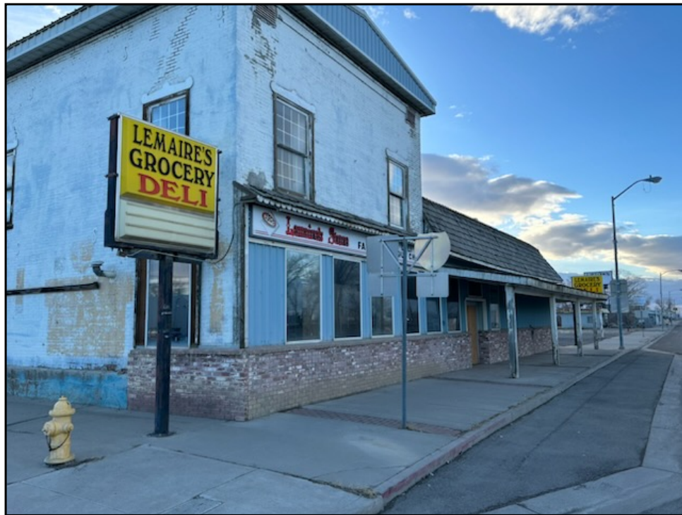
1 : View of Subject Property Exterior.
