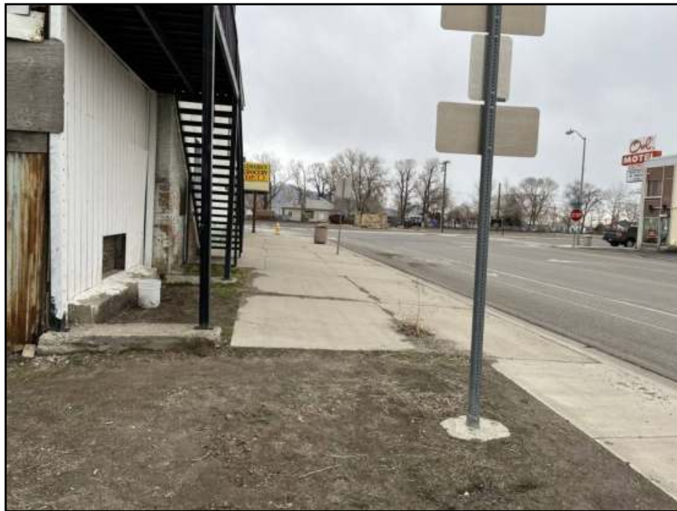
17 : View of the southeast side of the structure on the Subject Property.
