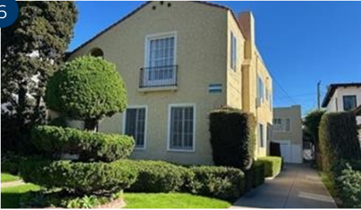
280 Park 280 Park Avenue, Long Beach, CA 90803
