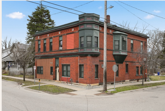
Exterior at the intersection of 3 rd St E & Forest St N
