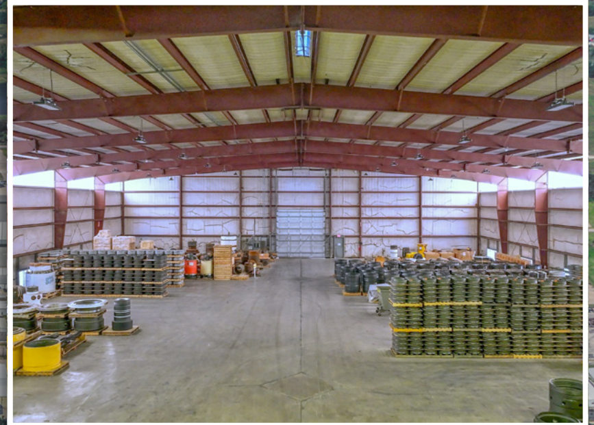
BUILDING A INTERIOR
