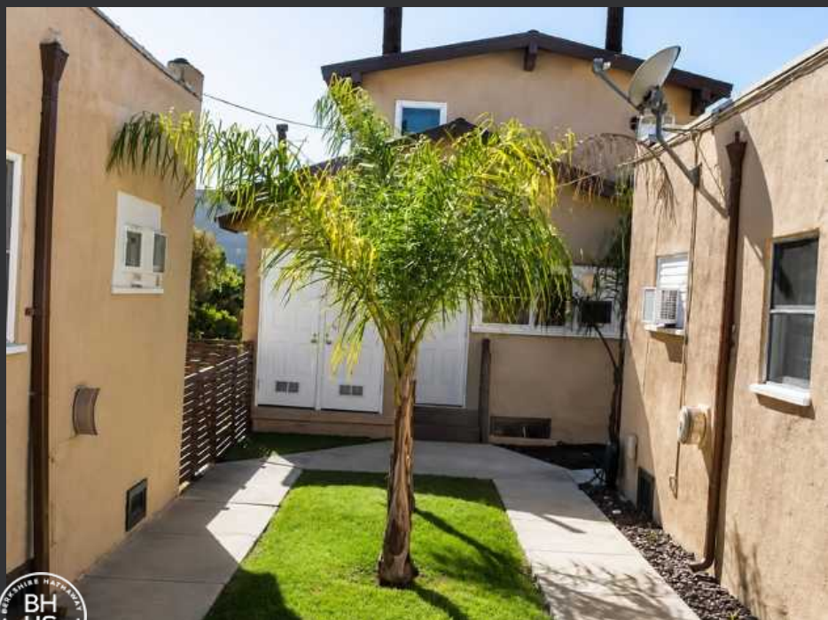
WALKWAY BETWEEN UNIT C & D
