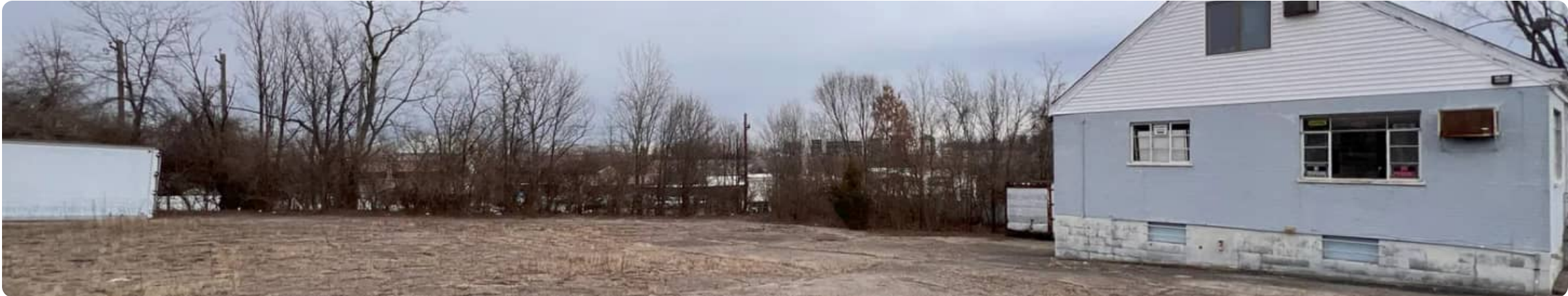
Ground Level — Side View
