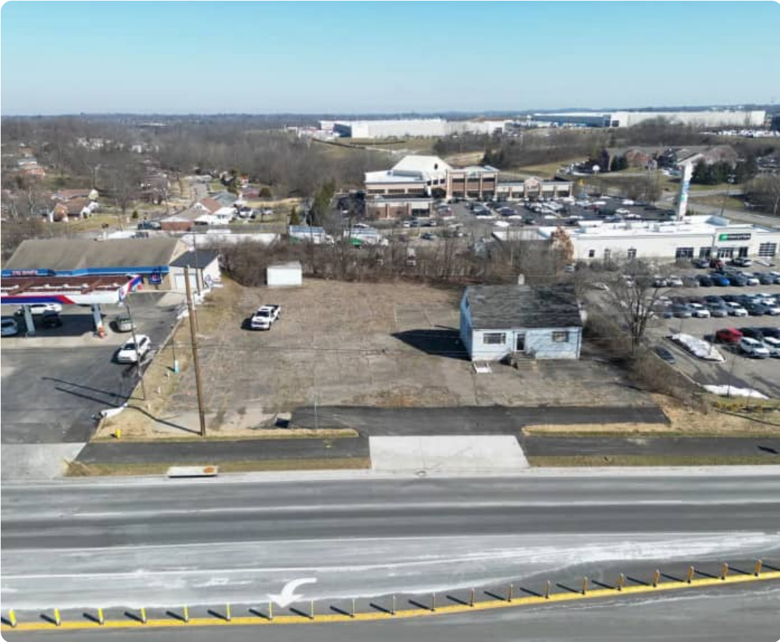
Donaldson Highway Frontage
