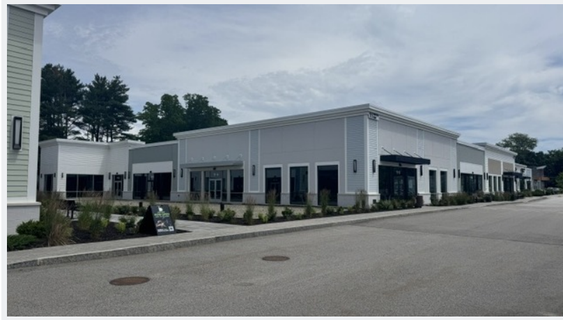
Building R3B — 11 Digital Way, Maynard, MA
