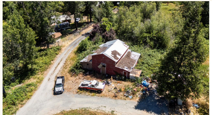
Existing improvements — residence and barn on R316942 (leased).
