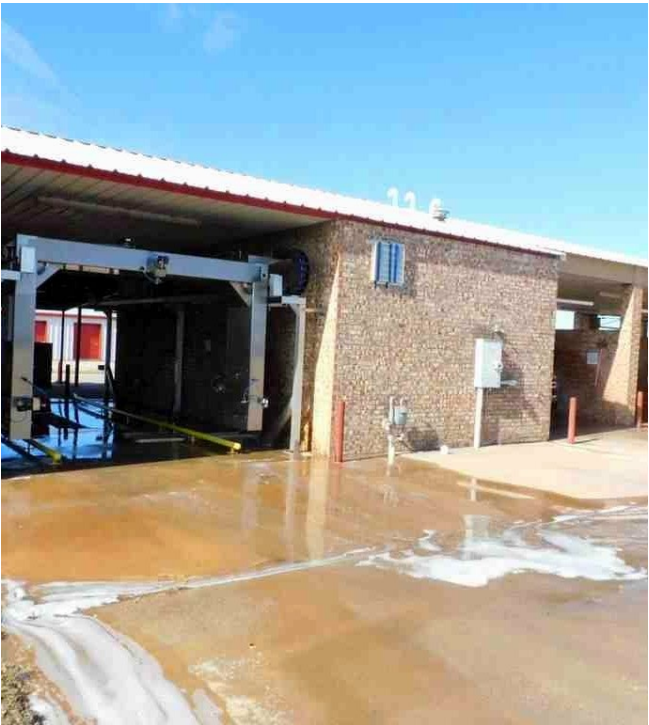
AUTOMATIC BAY & EQUIPMENT — SYSTEMS UPDATED ~2021
