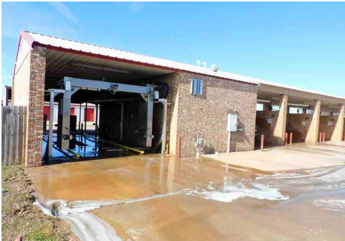
AUTOMATIC BAY — BRICK & METAL ROOF
