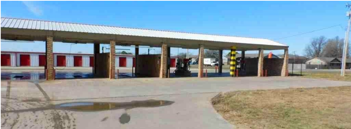
WASH BAYS AND COVERED VACUUM CANOPY — BRICK CONSTRUCTION WITH METAL ROOF
