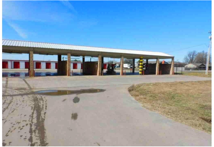
BAY LINEUP — EAST APPROACH
