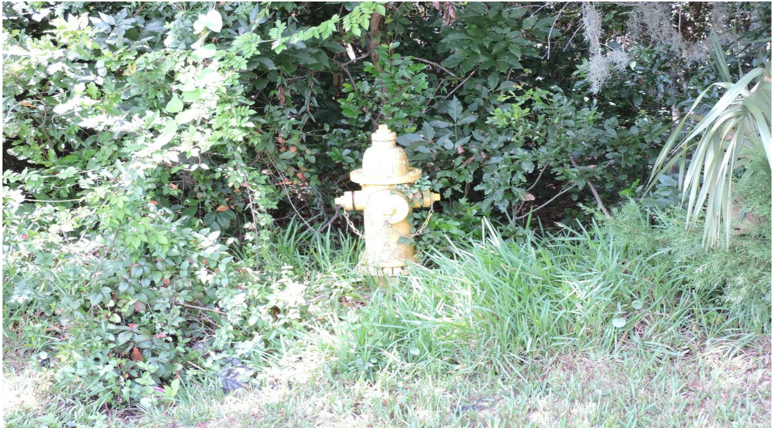
Water at Site
