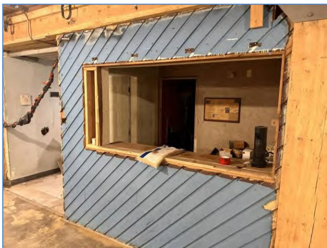
Basement Level: Bar area.
