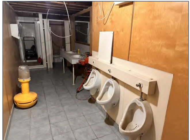
Basement Level: One of two partially finished bathrooms.
