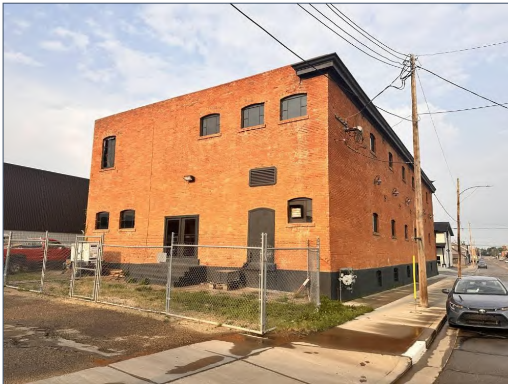
Northeast elevation (rear) of the Subject Property.
