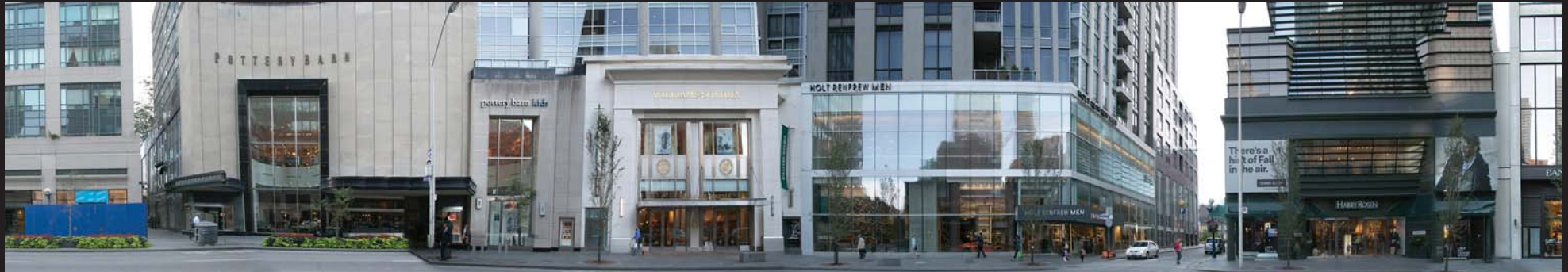
NORTH VIEW OF BLOOR STREET WEST
