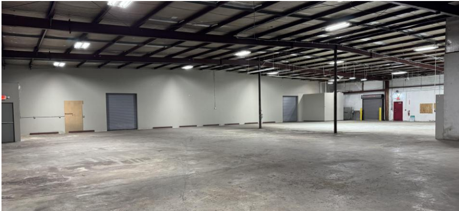
Suite B Warehouse — Interior View
