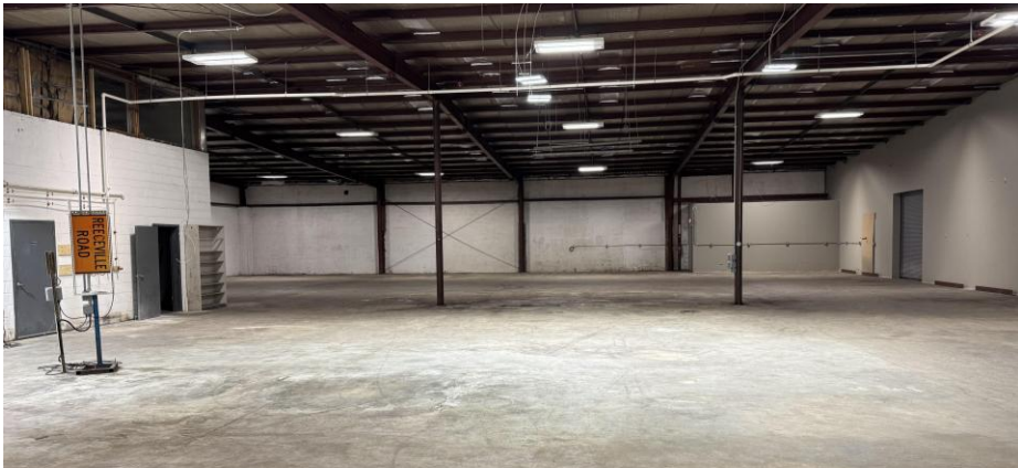
Suite B Warehouse — Interior View
