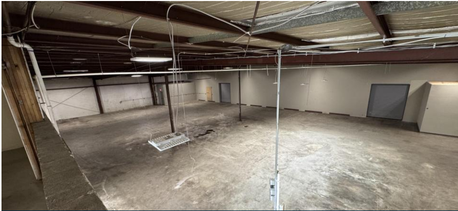
Suite B Warehouse — Interior View
