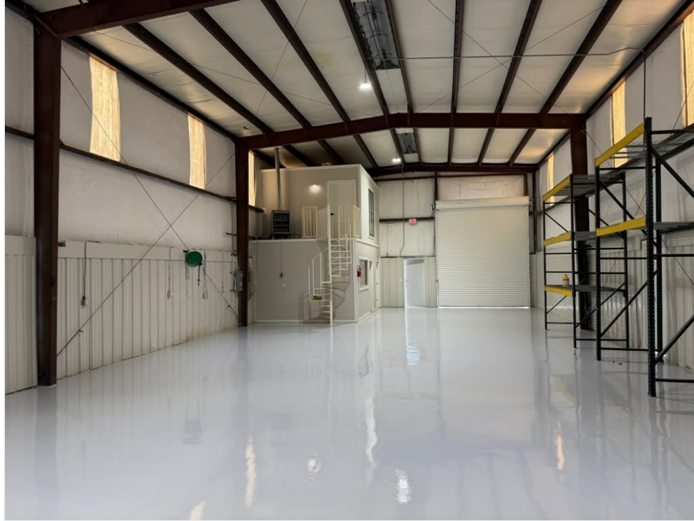
Inside of Warehouse
