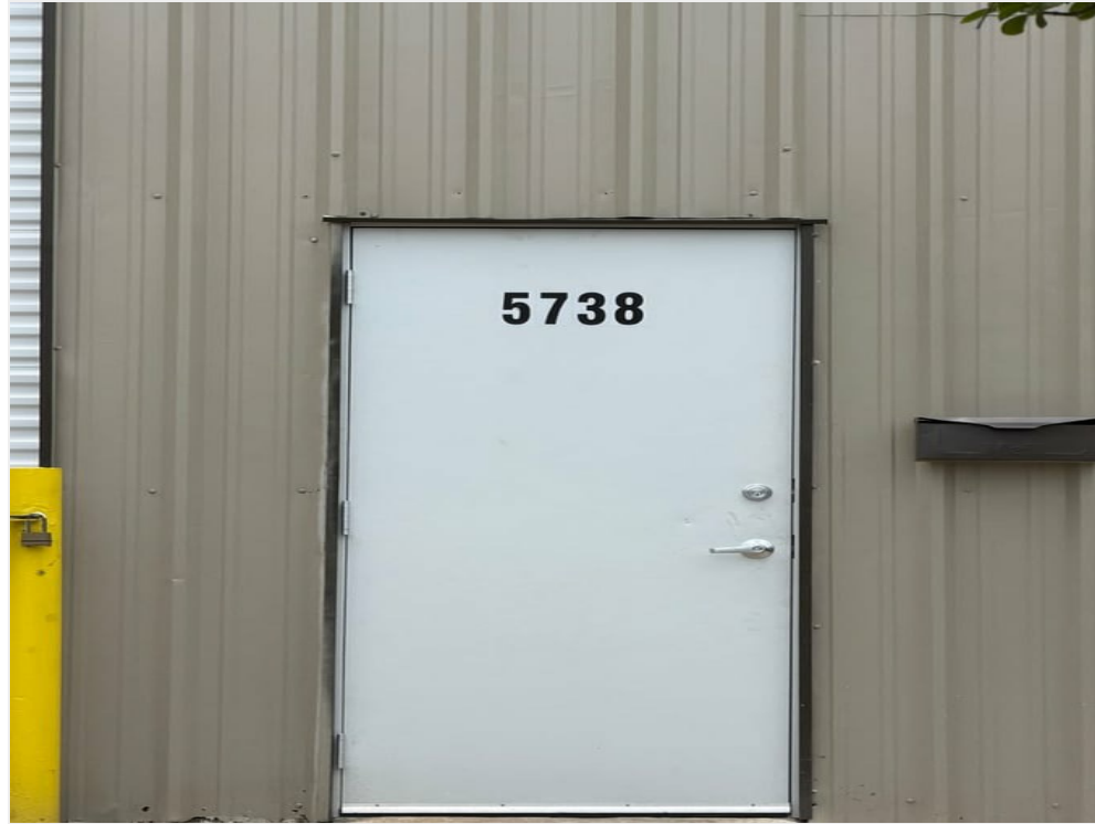
Door to the Warehouse
