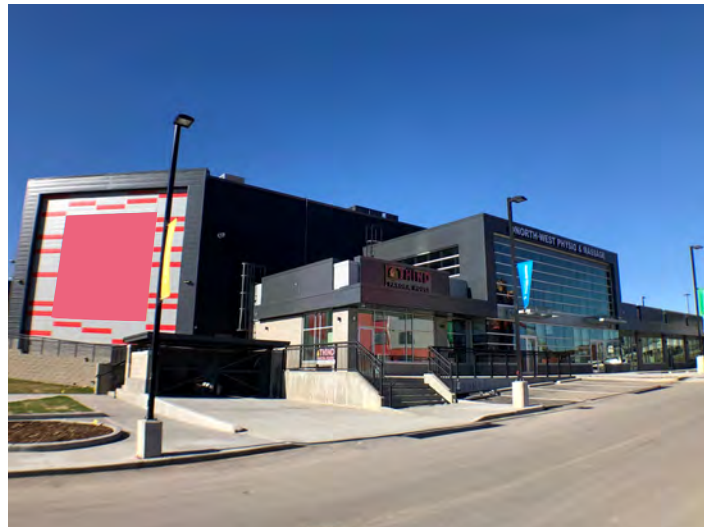
Building U - (Leased)
