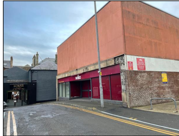
Entrance Unit 4B
