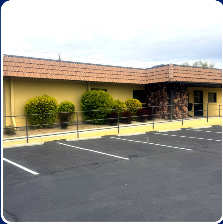
REAR OF BUILDING
