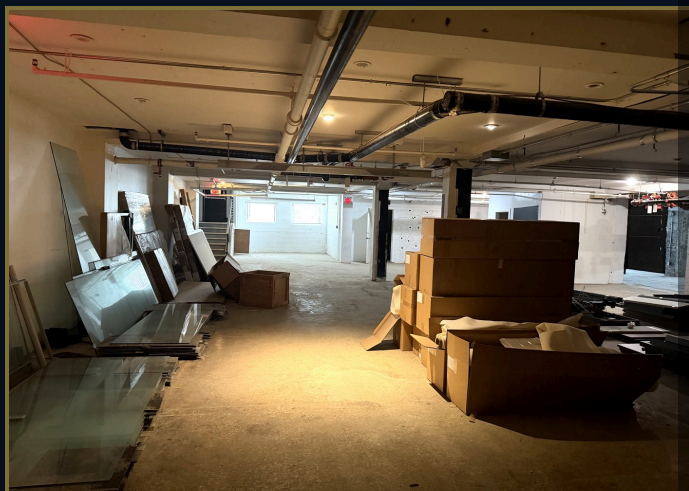
OPEN FLOOR PLATE · STAIR & DAYLIGHT BEYOND
