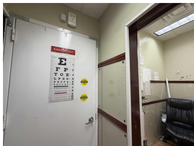
The lead-shielded radiology door — signage and regulatory standing in place
