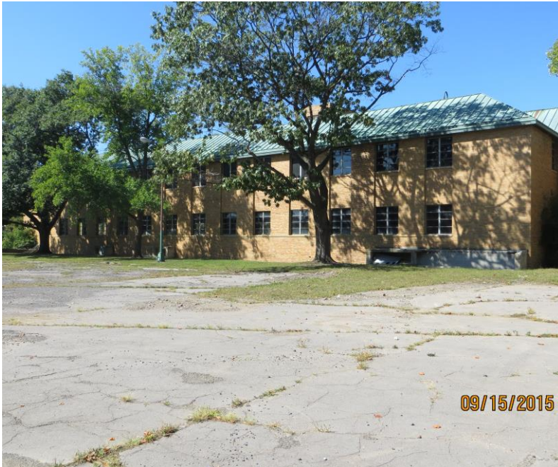
Partial view of building's east side
