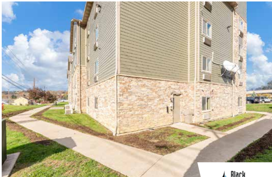
Access Around Building
