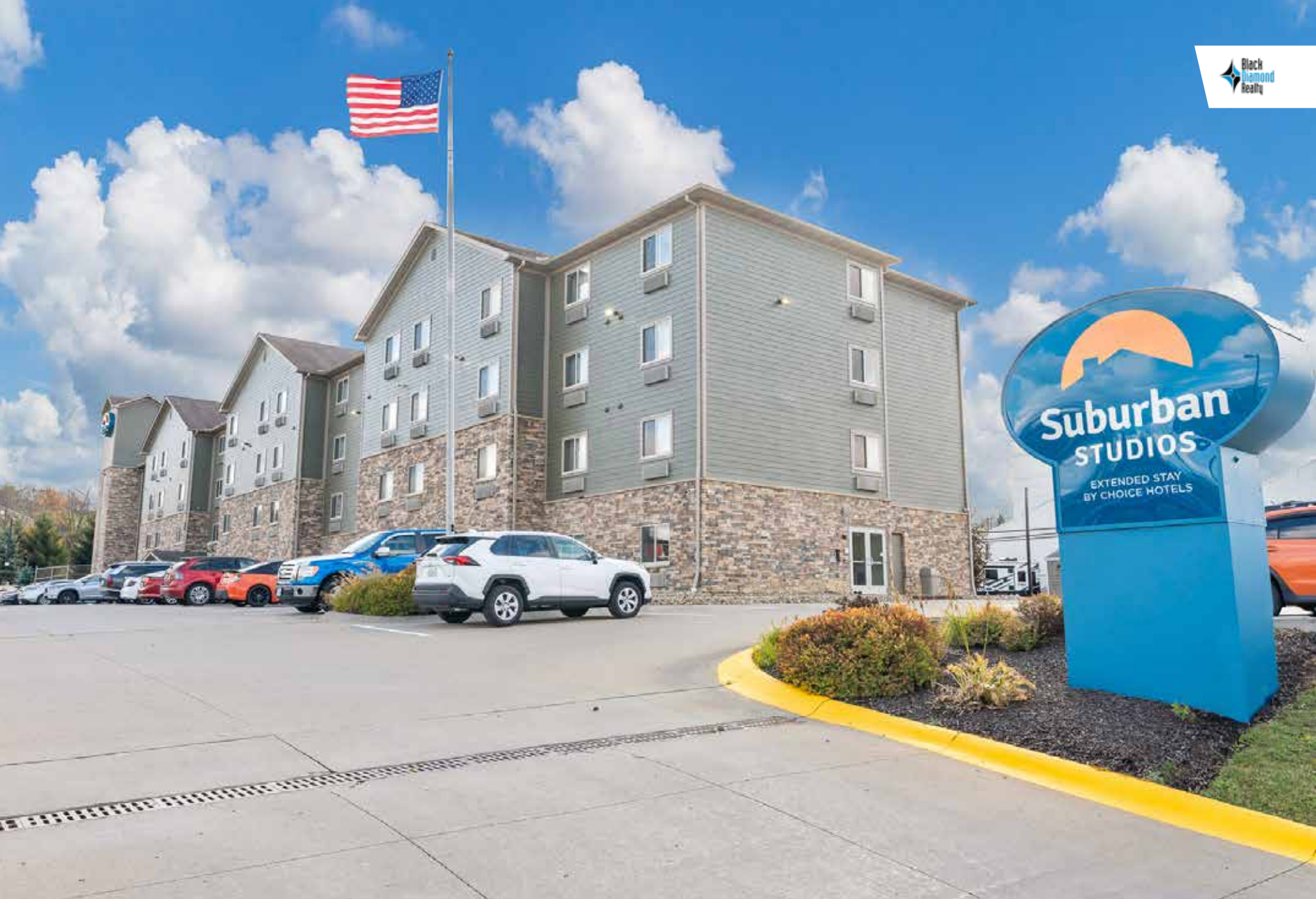
Parking Lot Entrance
