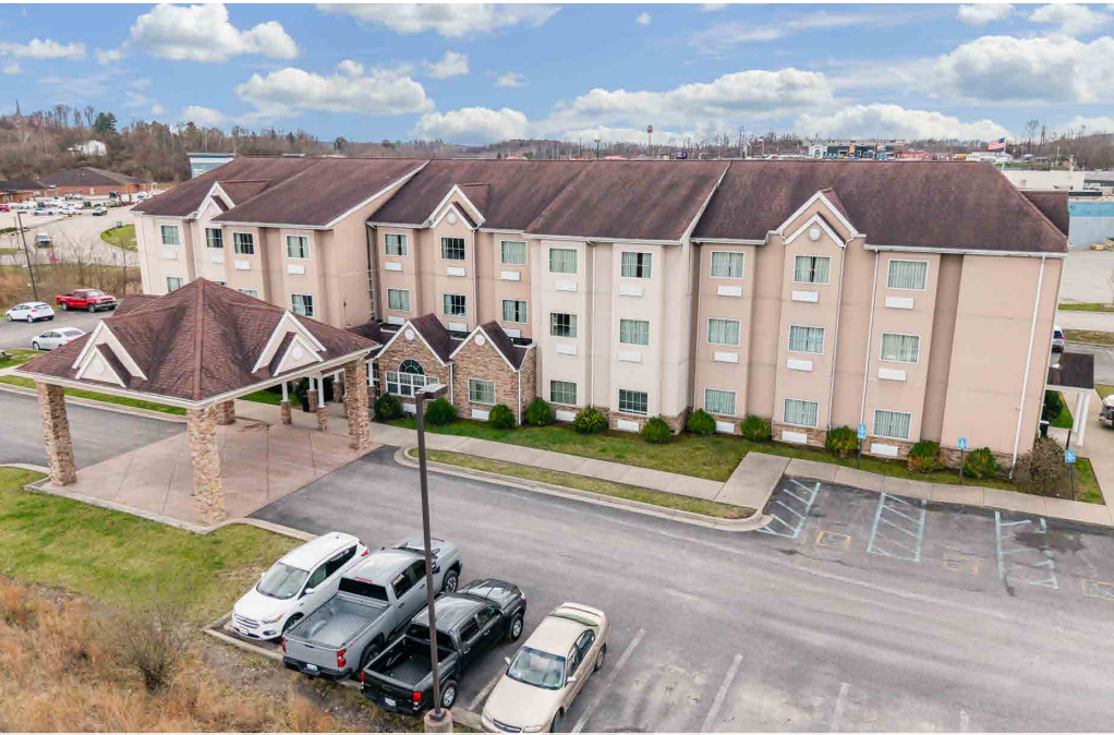
Aerial Facing South.
