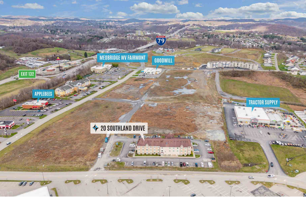
Aerial Facing Northeast.
