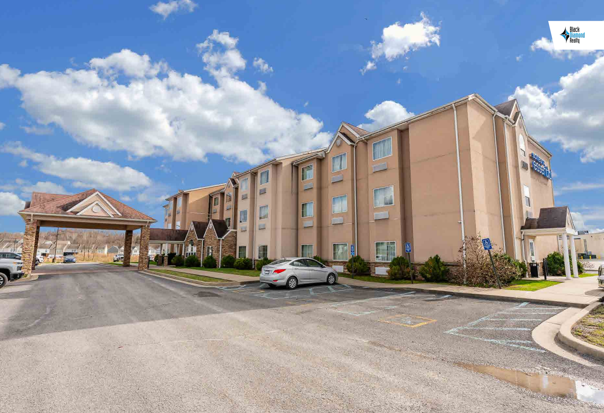
Parking Lot and Main Entrance.
