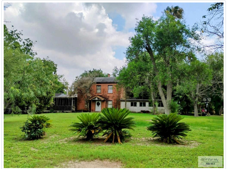
VIEW OF FRONT OF HOME
