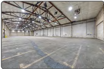
Bay 1: Northwest Corner
