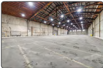
Bay 2: Southwest Corner
