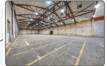
Bay 1: Southeast Corner
