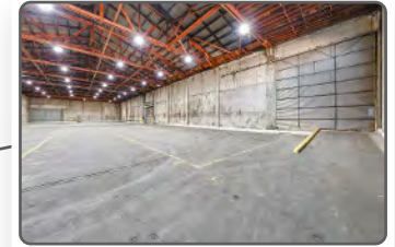
Bay 2: 17'x18' Dock Door
