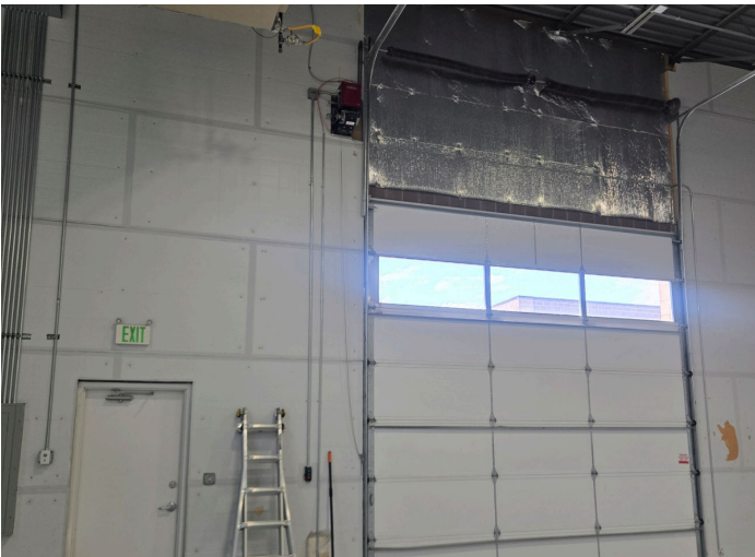
The 14' x 14' insulated ground-level door sits inside the main floor, with a gas unit heater above and a secondary man door alongside.
