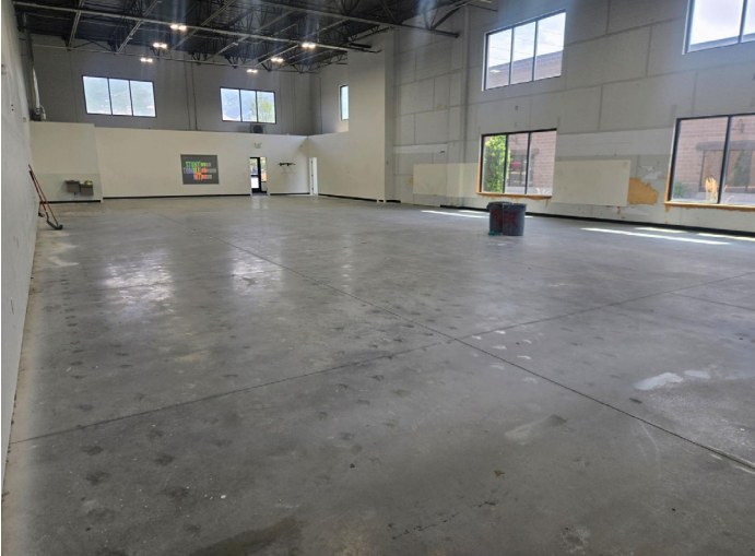
The open main floor — roughly 4,000 SF of clear-span space under 20' ceilings, with clerestory windows on two walls filling the room with natural light.
