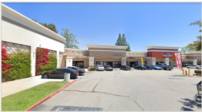
Storefronts on the west building
