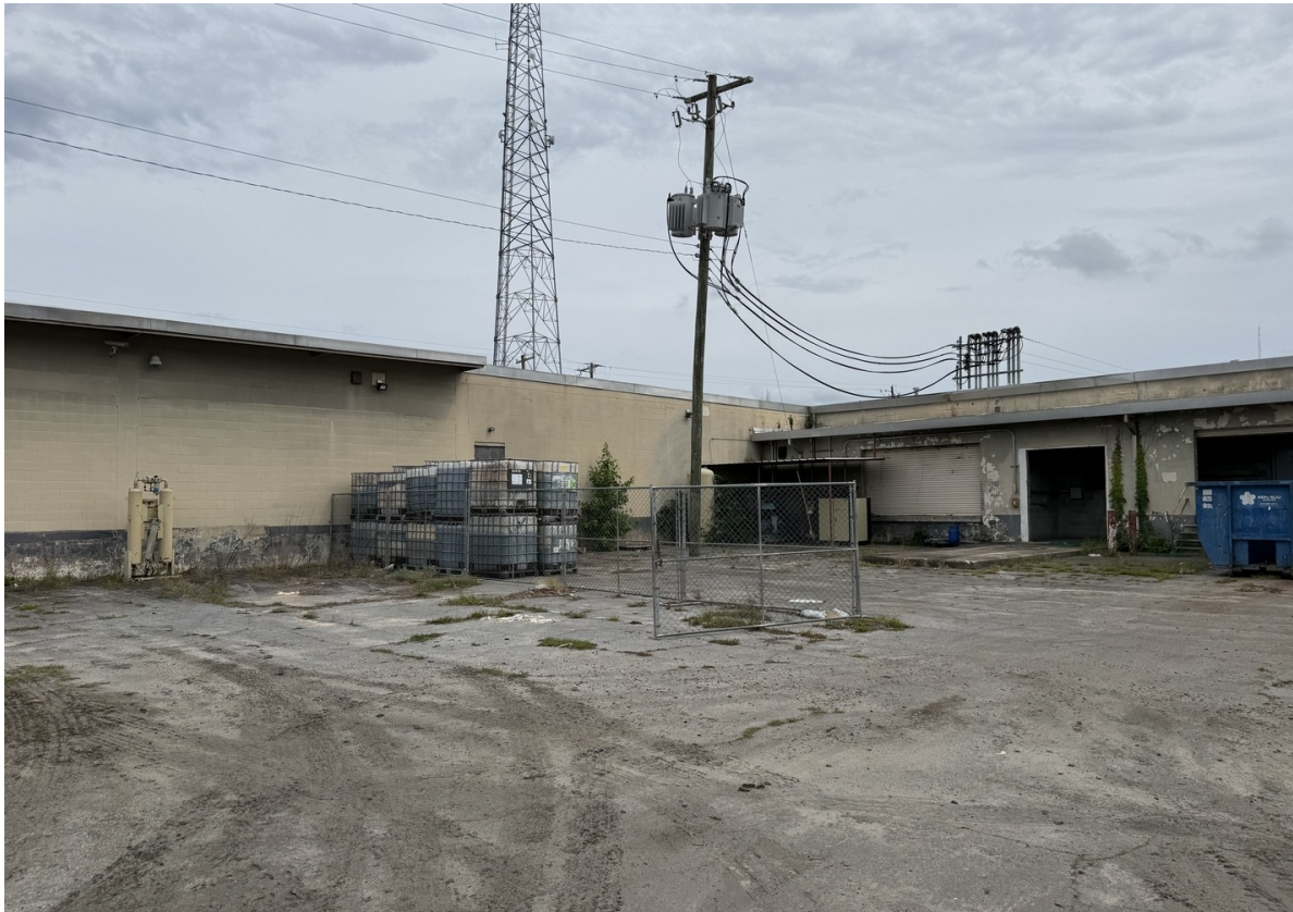
OUTSIDE STORAGE / YARD AREA
