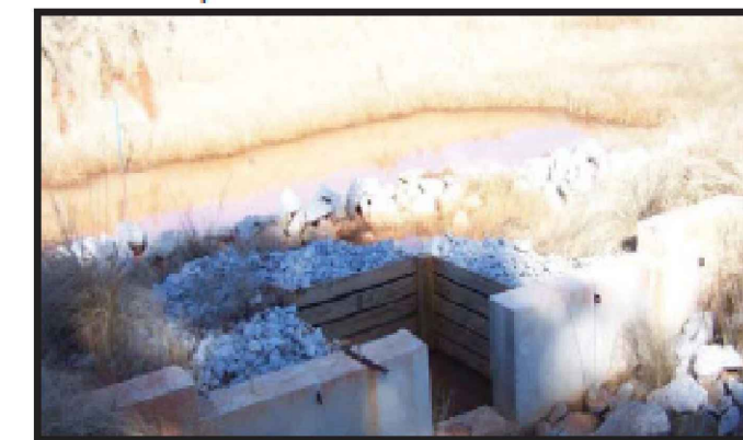
Example of Slotted Board Dam
