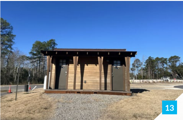
BATH & SHOWER FACILITY
