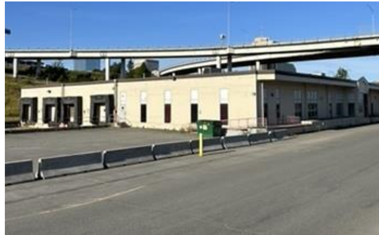
Building 4 – View from East
