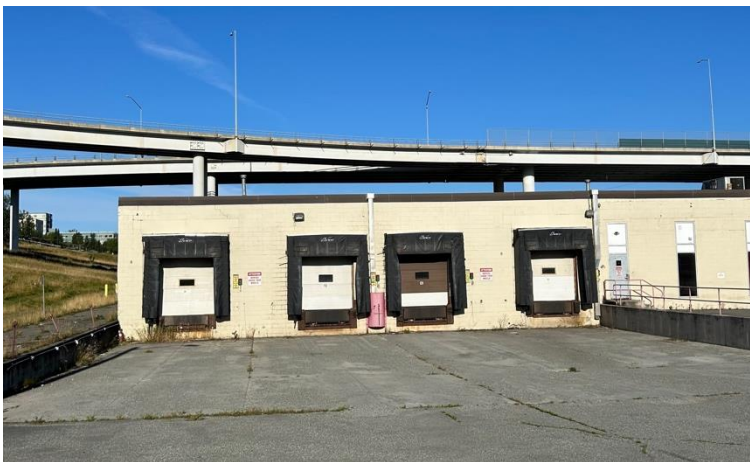
Building 4 – Dock Doors
