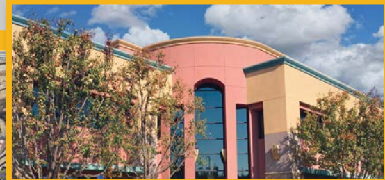
1502 Mill Rock Way
