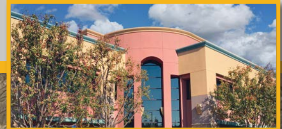
1502 Mill Rock Way
