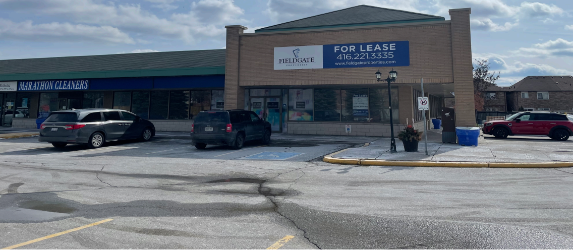
HUMBERLAND FRONTING EXTERIOR FACADE SIGNAGE
