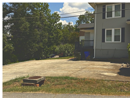
On site parking behind the building
