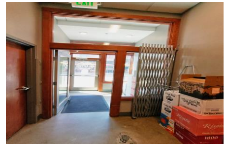
Secondary entry with retractable security gate
