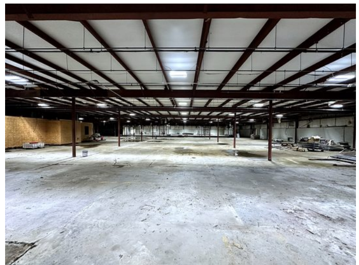
Interior — clear-span structure
