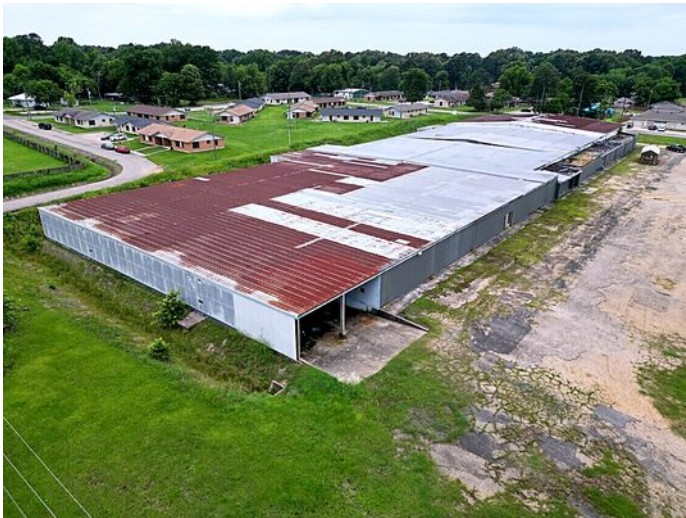
Aerial — covered loading end
