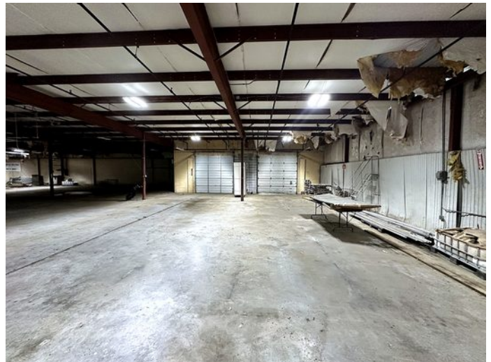
Interior — overhead loading doors
