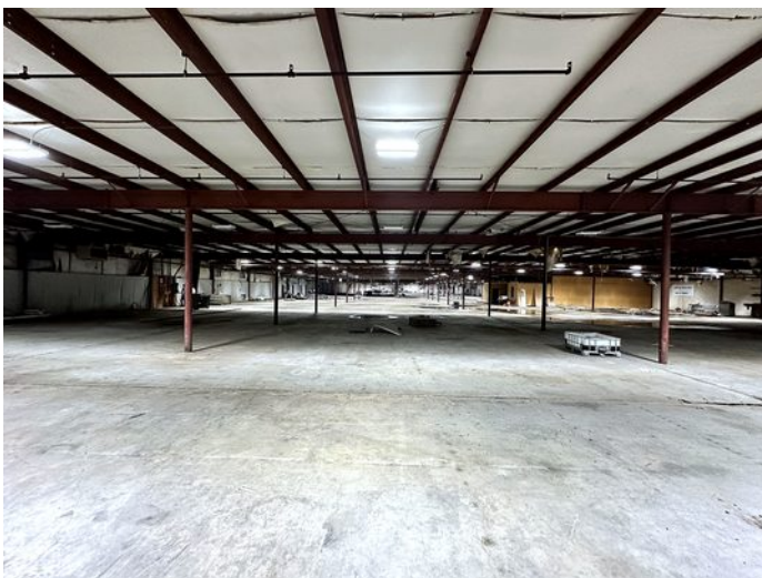
Interior — clear-span, dry floor
