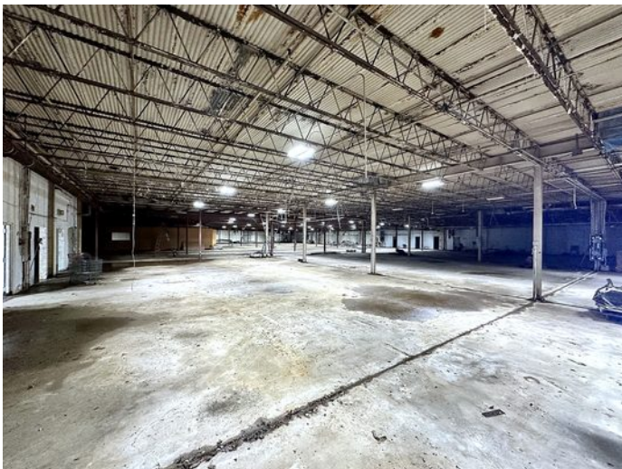
Interior — older section
