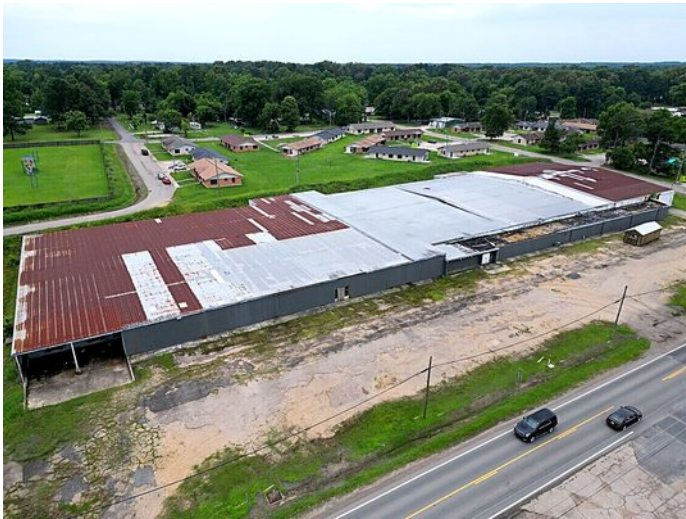
Aerial — building & road frontage
