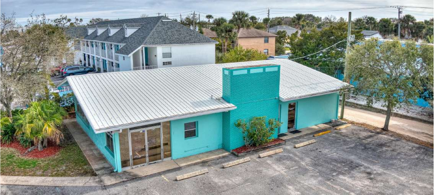
Concrete block construction. Metal roof.
