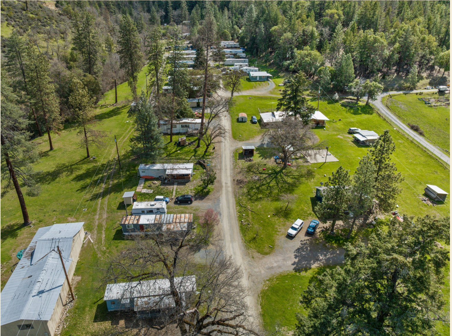
Park overview — manufactured homes, stick-built residences, and internal road network with mature trees along the eastern boundary.
