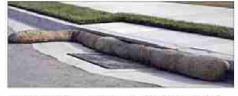
STRAW WATTLE INLET FILTER PROTECTION
