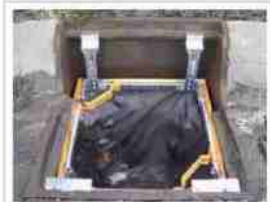
FLEXSTORM INLET FILTER PROTECTION
