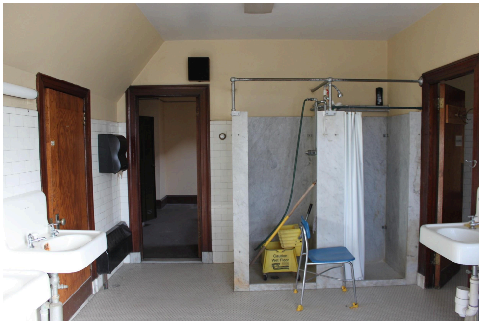
Figure 21. Historic fixtures in second story bathroom.
