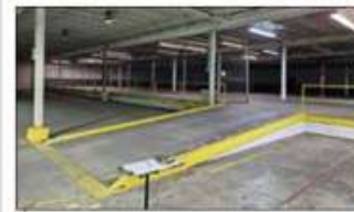
8 INTERIOR VIEW A2
