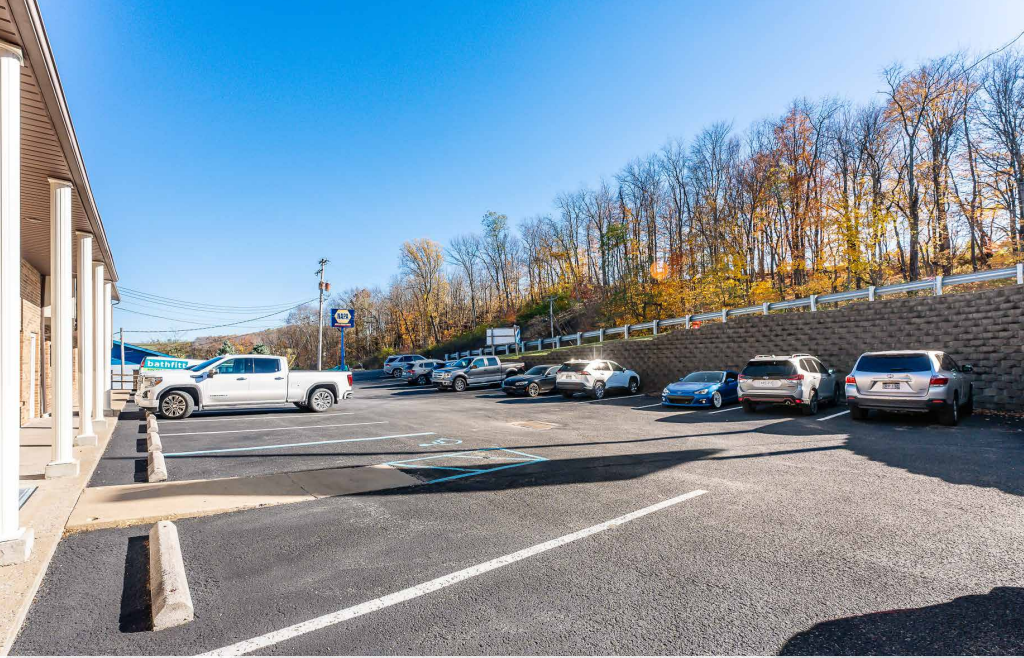
Exterior Front Parking Lot
