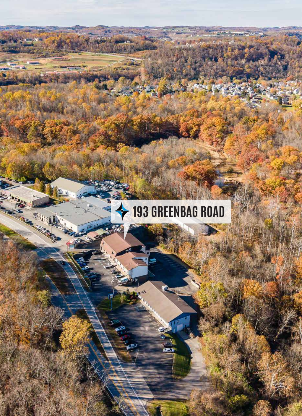
Aerial Facing West.
