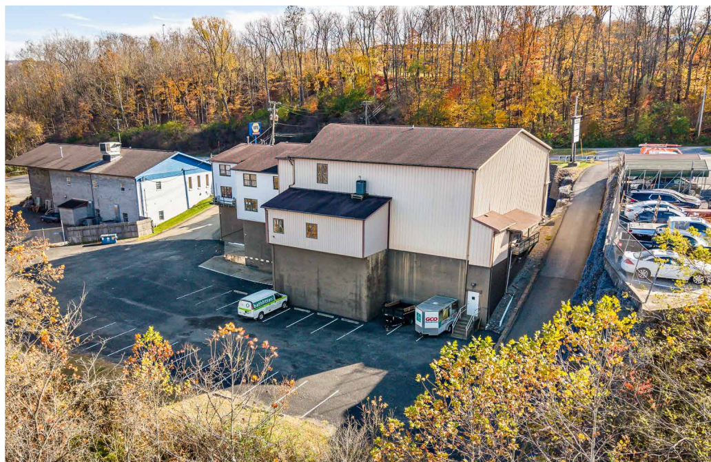
Aerial Facing South.
