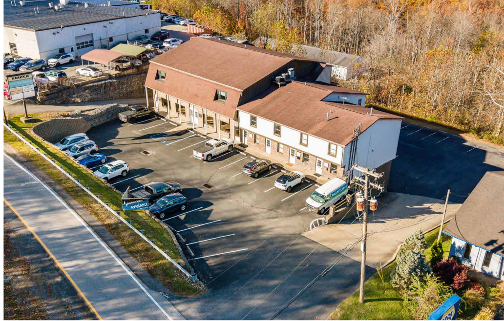
Aerial Facing Northwest.
