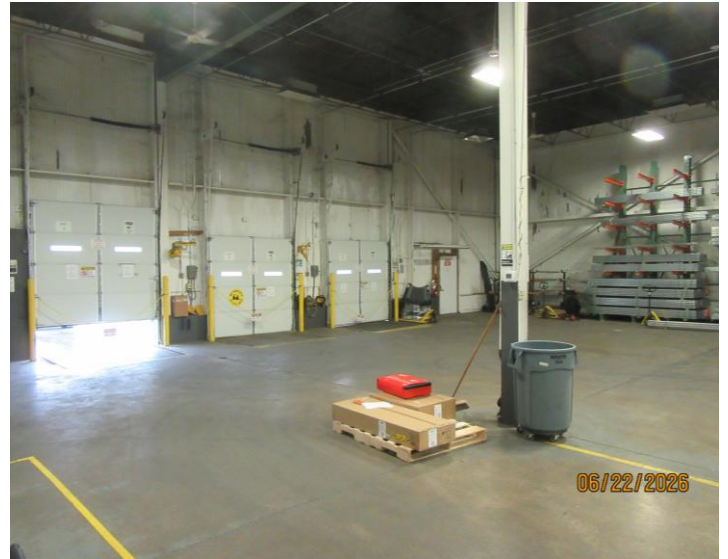
Three (3) Dock Doors with Levelers
