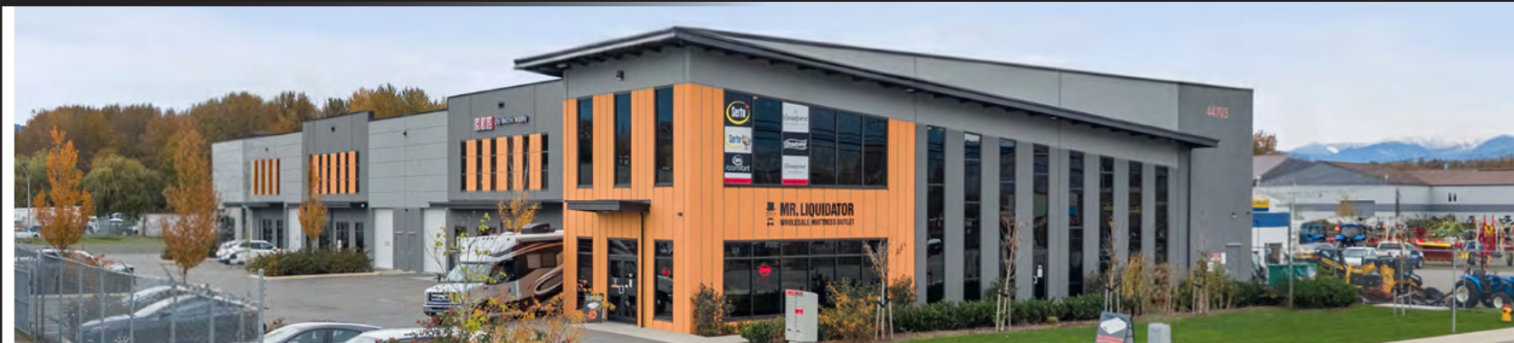
YALE ROAD BUSINESS PARK 44703 Yale Road, Chilliwack, B.C.
