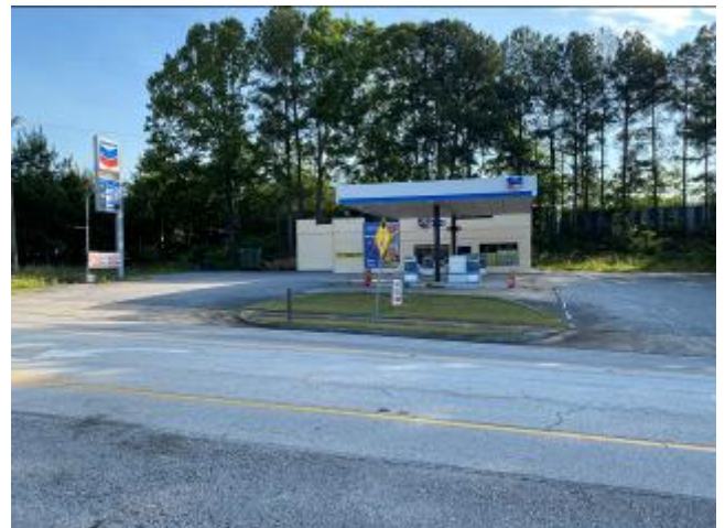
View facing north of the adjoining gas station beyond Mize Road.
