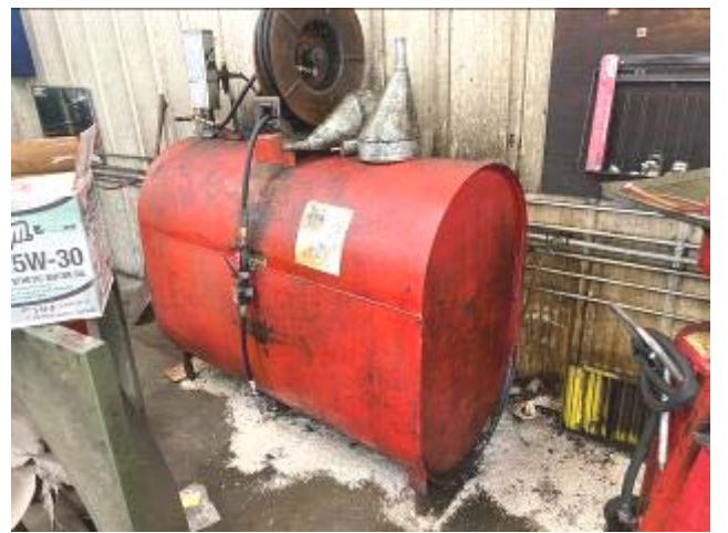
Three hundred-gallon waste oil AST with observed staining and absorbent along the southern wall of the automotive garage.
