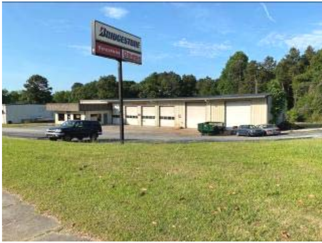
View of the former Casey's Pro Tire facility located on the subject property. View facing southeast.
