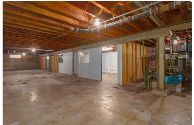
Concrete basement — bulk-storage tier.
