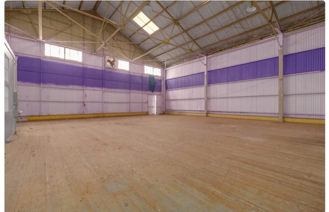
Warehouse zone — skylit, high-clearance industrial space.
