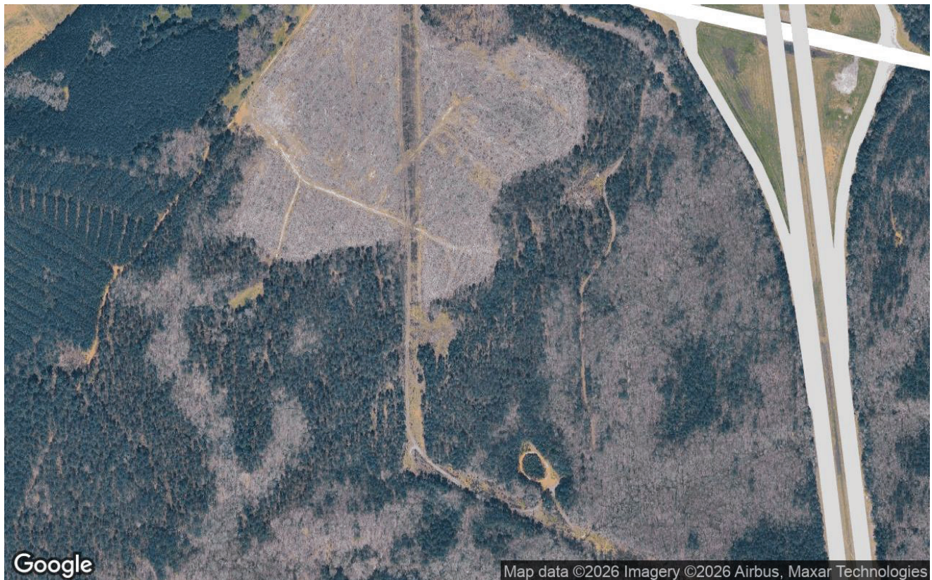
Existing conditions aerial showing terrain pattern, cleared areas, and physical site context near the interchange.
