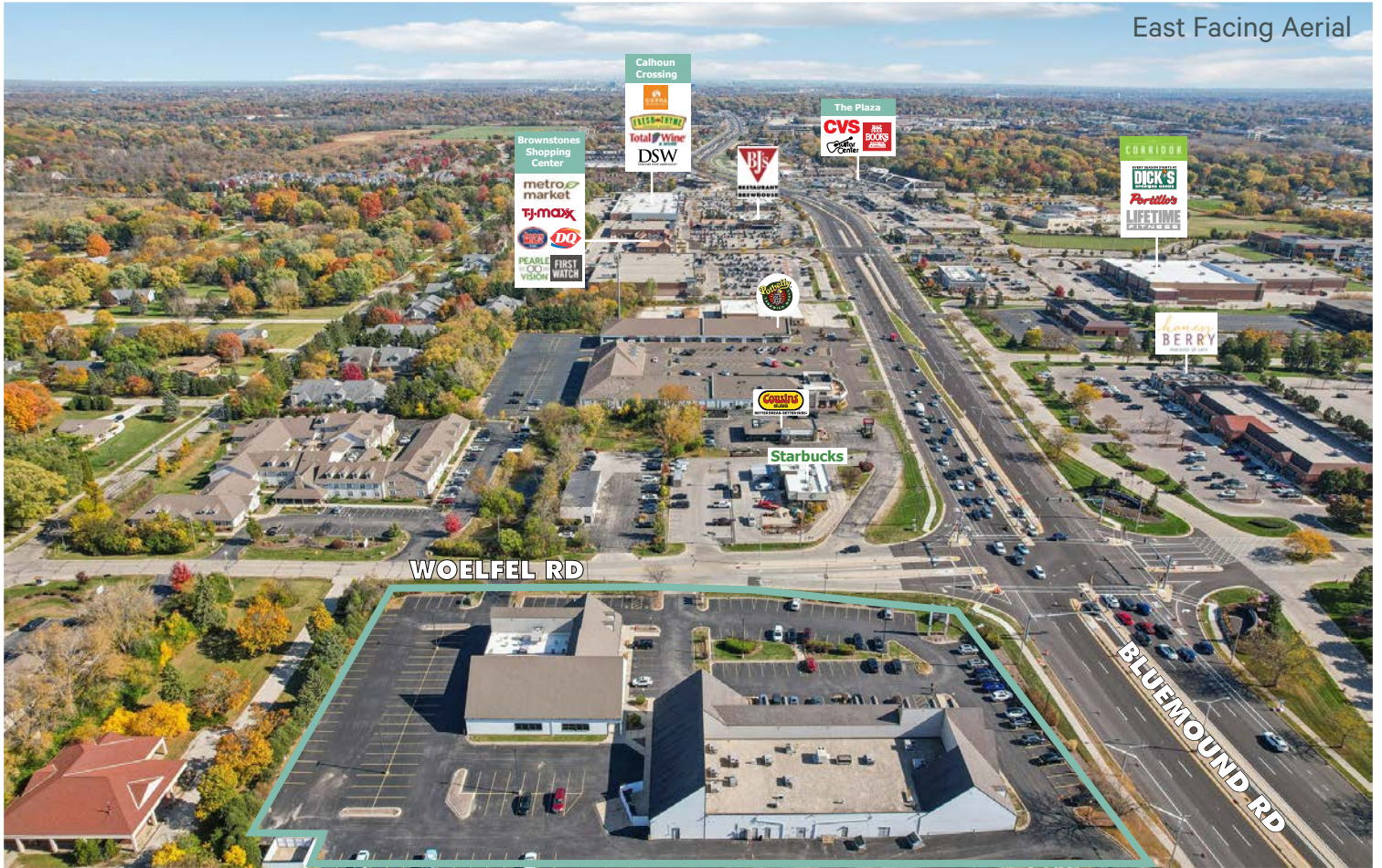
West Facing Aerial
