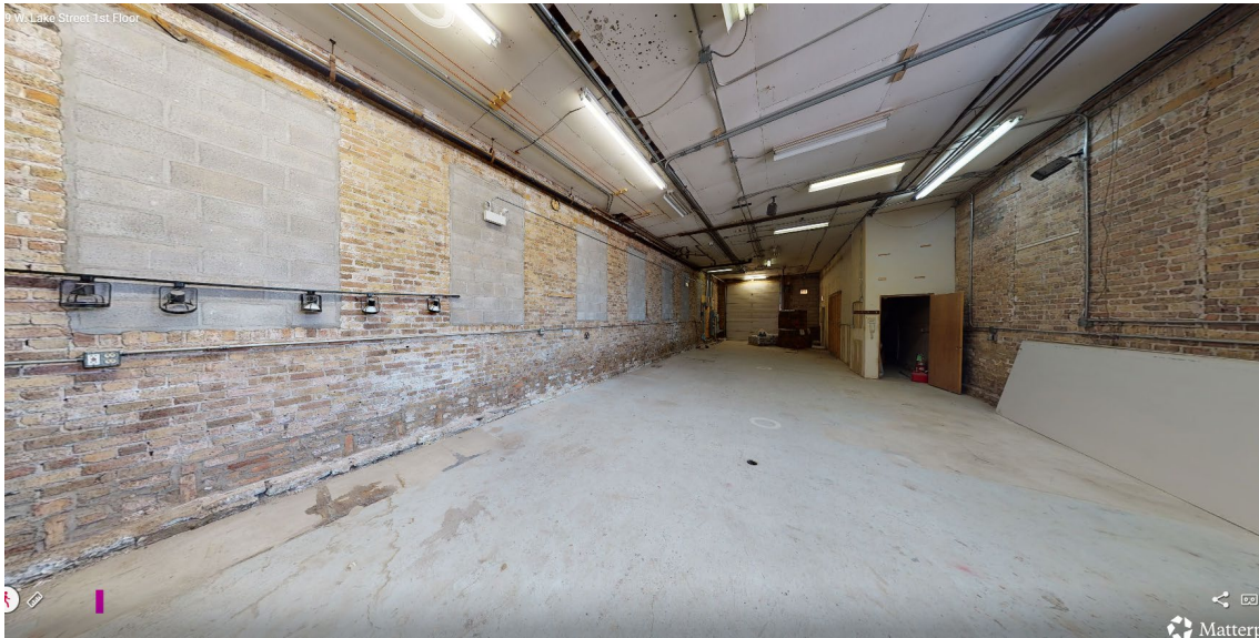
Rear area of building interior, loading door off the alley.
